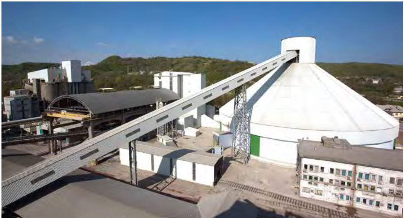
Conveyor belt of the new clinker silo
